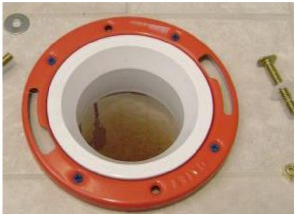
**8.6.2.4.2** If the flange was in good condition when the original toilet was removed, it may have been left on the floor. If the flange looks cracked or worn, replace it.
